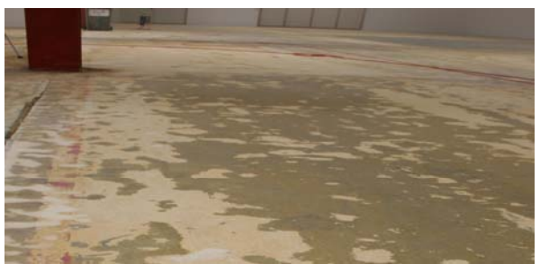
Removal of old coatings
