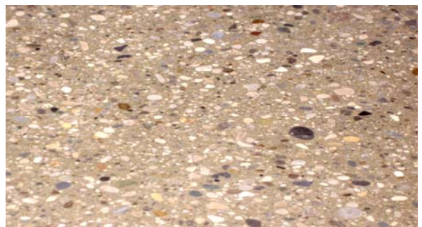
Concret polishing
