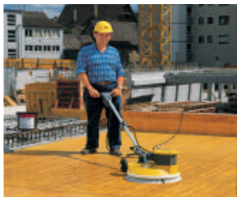
Scrubbing, cleaning and sealing
