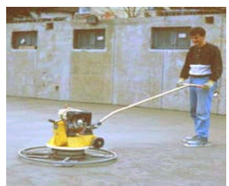
Trowelling of concrete with electrical or gasoline type
