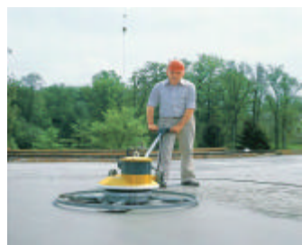
Trowelling of concrete with electrical or gasoline type
